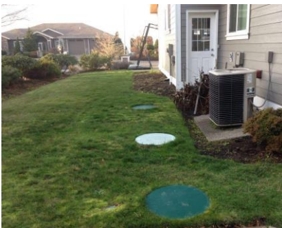
Yard nicely landscaped with the lids camouflaged in. Grass is the best groundcover for all septic components.
