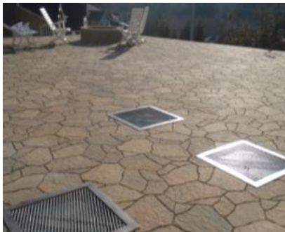
This natural flag stone patio that still provides access to your septic tank covers and can be removed for extensive work.
