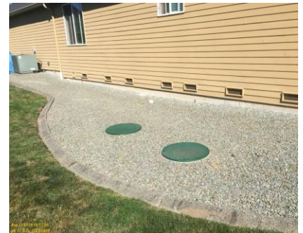
Gravel is another alternative coverage for your septic system especially when placed in a pathway.
